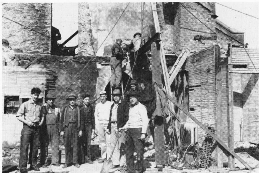
It was on Good Friday when the Scovill photographer chanced by the ruins of the Mill Plain Union Church and found this group of Scovillites helping to clean up debris in preparation for reconstruction. Besides working that day off, they've been generously contributing spare hours after work helping out. Above, left to right, are Les Coley, Jr., West Machine; Lee Garrigus, Carpenter Shop; George Aitchison and Jerry Cepelak of Machine Tool Room, 112 Building; Elbert Coley, Oil House; Les Coley, Sr., General Stores; and Maynard Rogers of Auditing.
